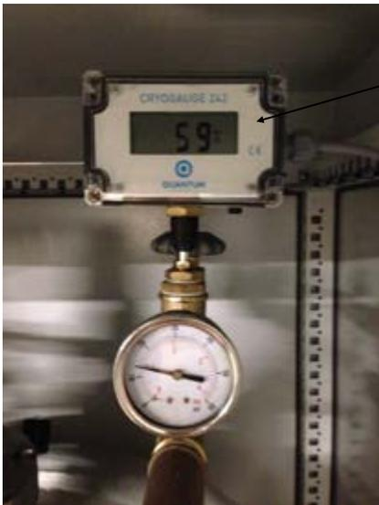
LEVEL DISPLAY, IS ALSO SHOWN ON THE MAIN HMI SCREEN.
